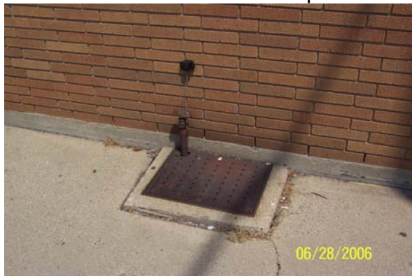
DT 59 – Potential UST Vent Pipe
